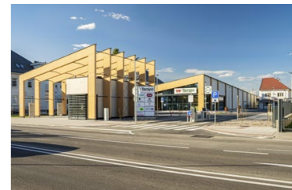
52 Retail park COOP Jednota NOVOSTAVBA
