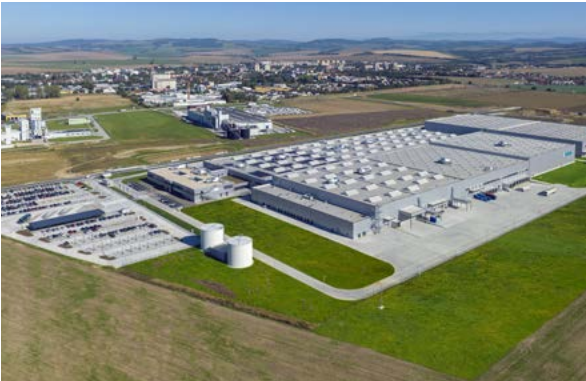
26 Vaillant Heat Pump Plant NOVOSTAVBA
